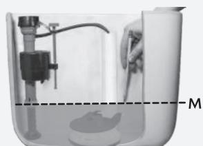
c) Remove old flapper. Install new flapper. Attach chain to flush lever with minimal slack.
